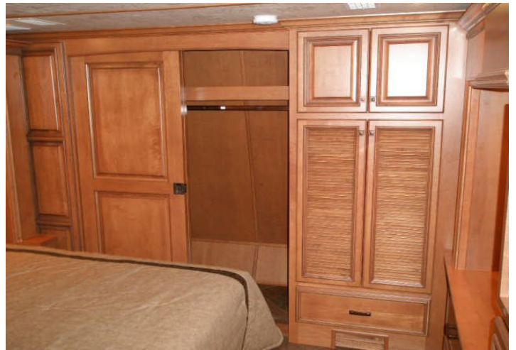
20 - Raised Panel Doors in Wardrobe
